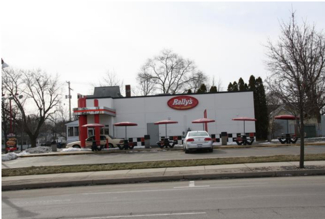
SOUTH – Commercial adjacent to south of site Southeast corner of Columbus Ave and Madison Ave Facing south from Columbus Avenue
