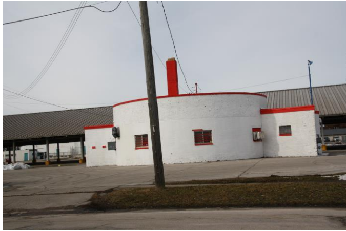
WEST – Commercial adjacent to west of site Chuckie's Market Restaurant Facing west from Jefferson Street Flea Market is structure behind restaurant
