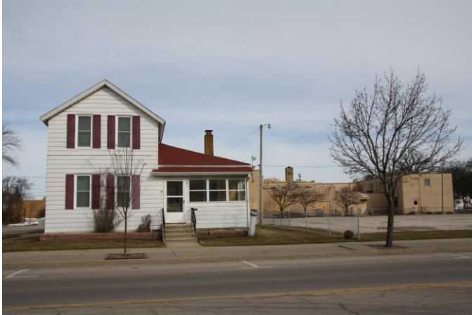
SITE – Columbus Avenue Apartments 501 Columbus Avenue, Bay City, MI Existing structures on site Facing north from Columbus Avenue
