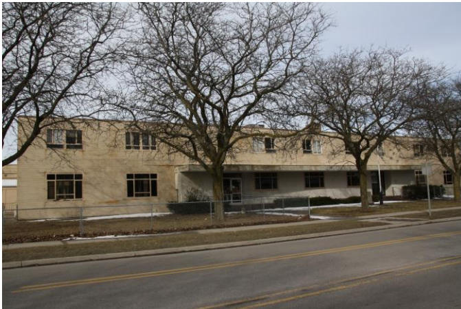
SITE – Columbus Avenue Apartments 501 Columbus Avenue, Bay City, MI Existing YMCA building on site Facing west from Madison Avenue
