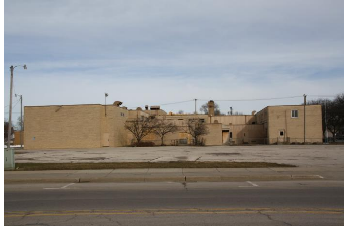
SITE – Columbus Avenue Apartments 501 Columbus Avenue, Bay City, MI Existing YMCA building on site Facing north from Columbus Avenue
