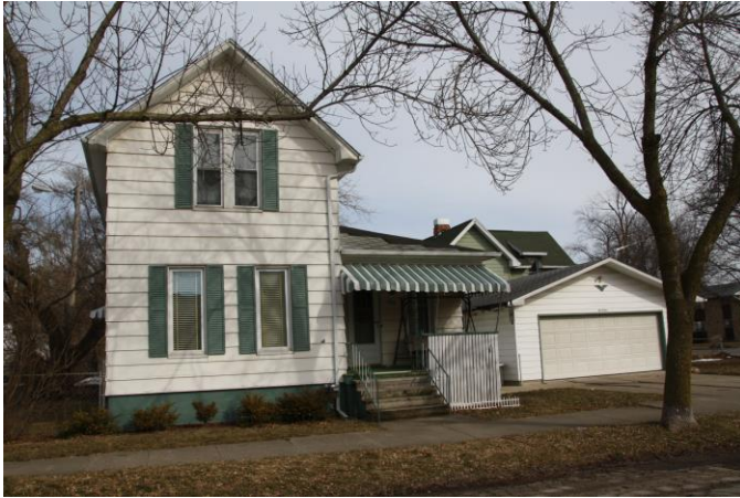
NORTH – Single-family home adjacent to north of site Northwest corner of Madison Ave and 11 th Street Facing north from 11 th Street
